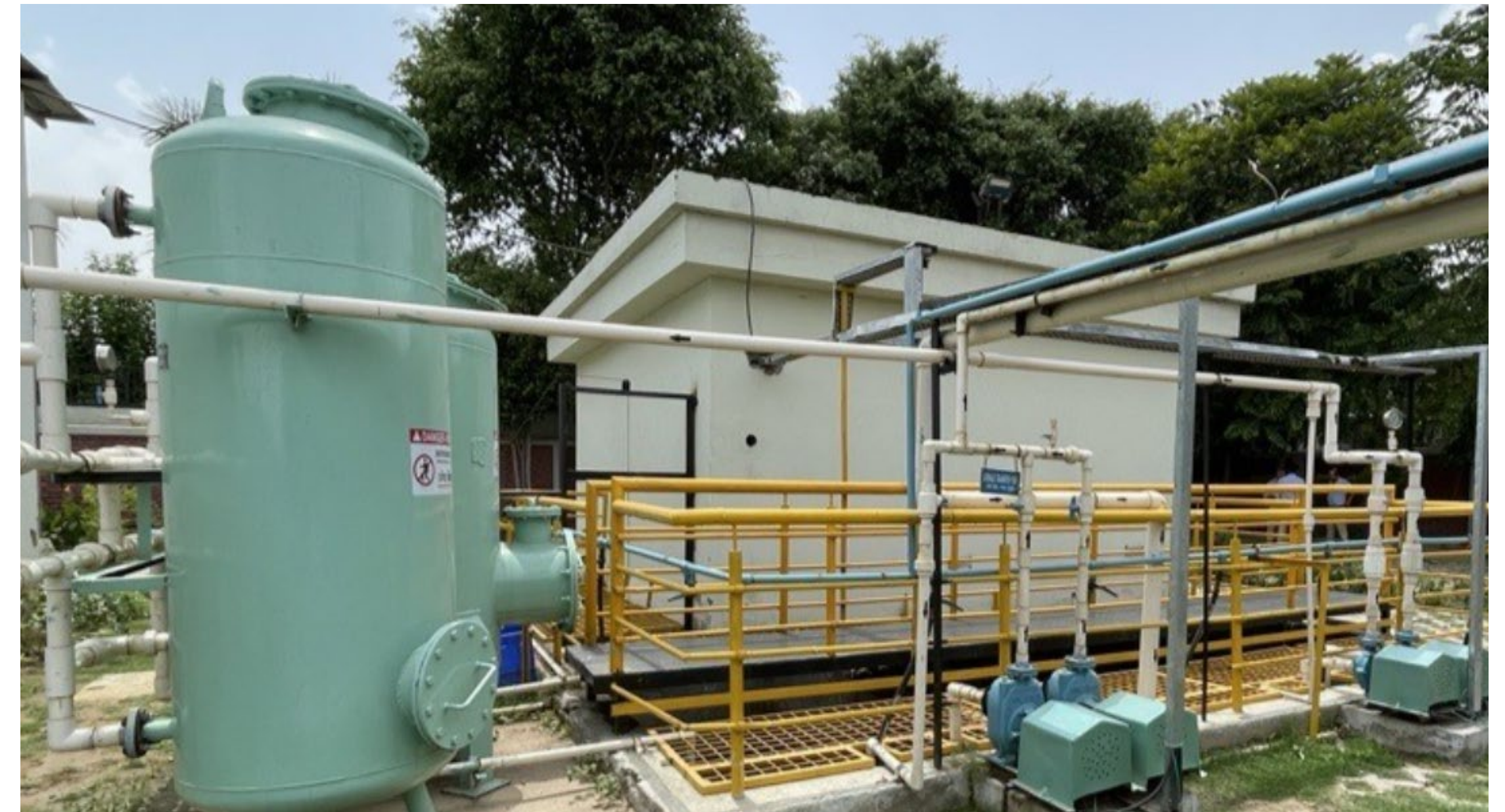
Water treatment plant in Bawal, India
